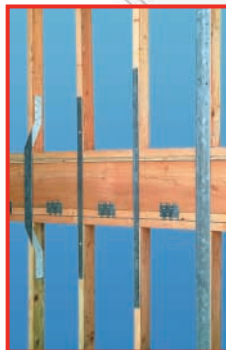
TYPICAL FLOOR-TO-FLOOR CONNECTIONS Pages 37 to 41, 148 to 153
